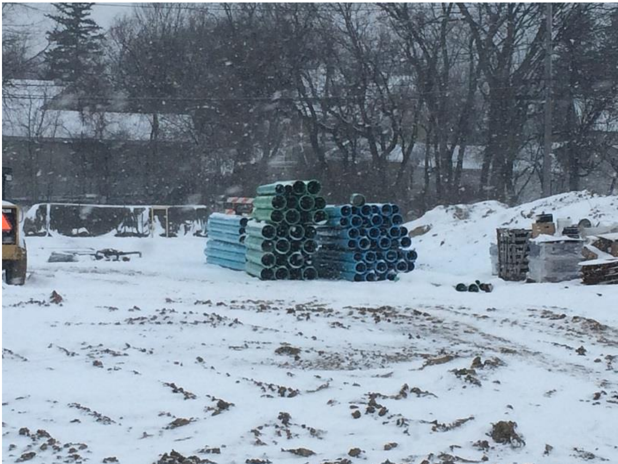
Site Utility Materials being delivered.
