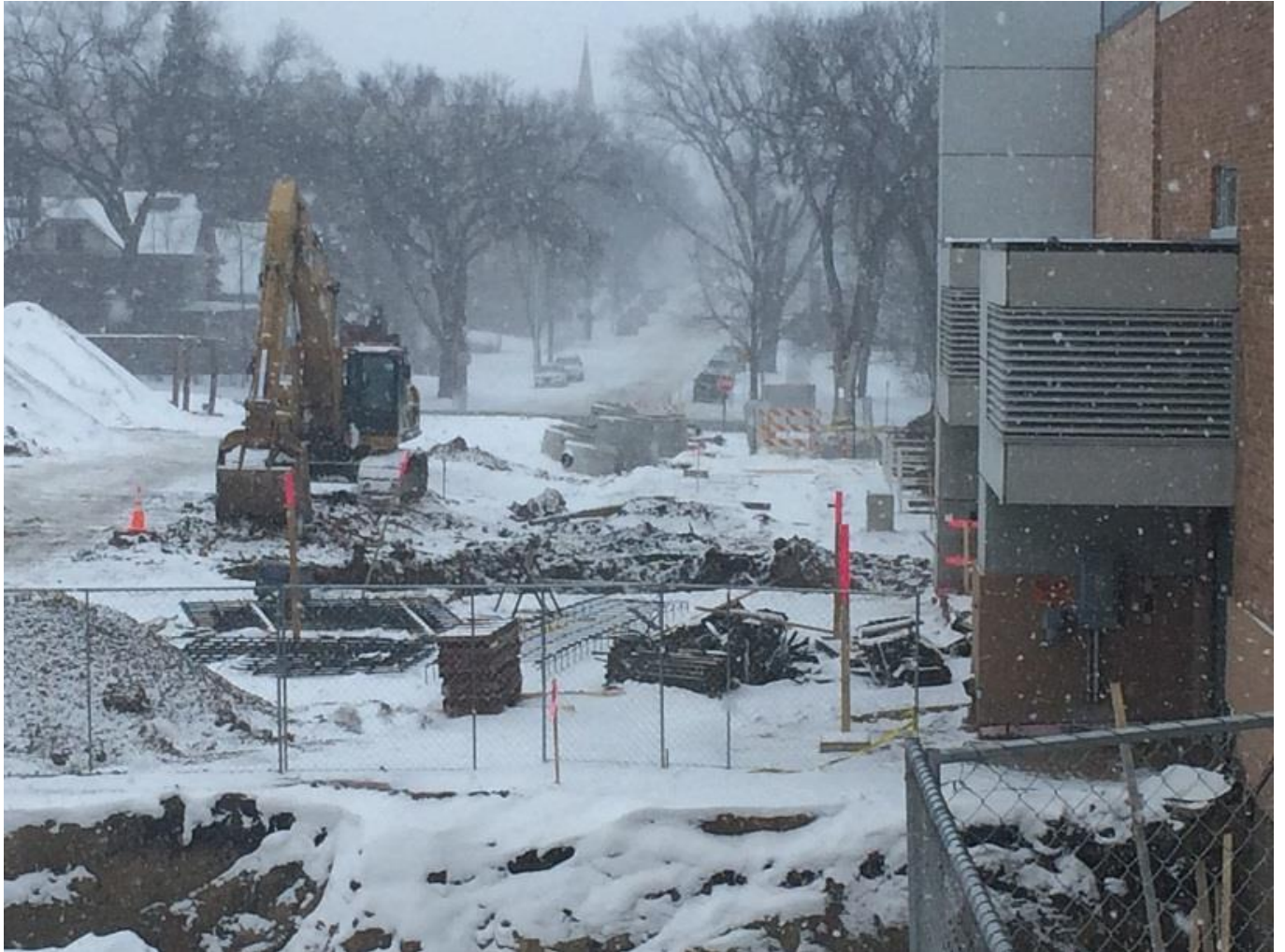
Site Utility Contractor working on Receiving Pit for boring rig and locating exact locations of existing utilities.
