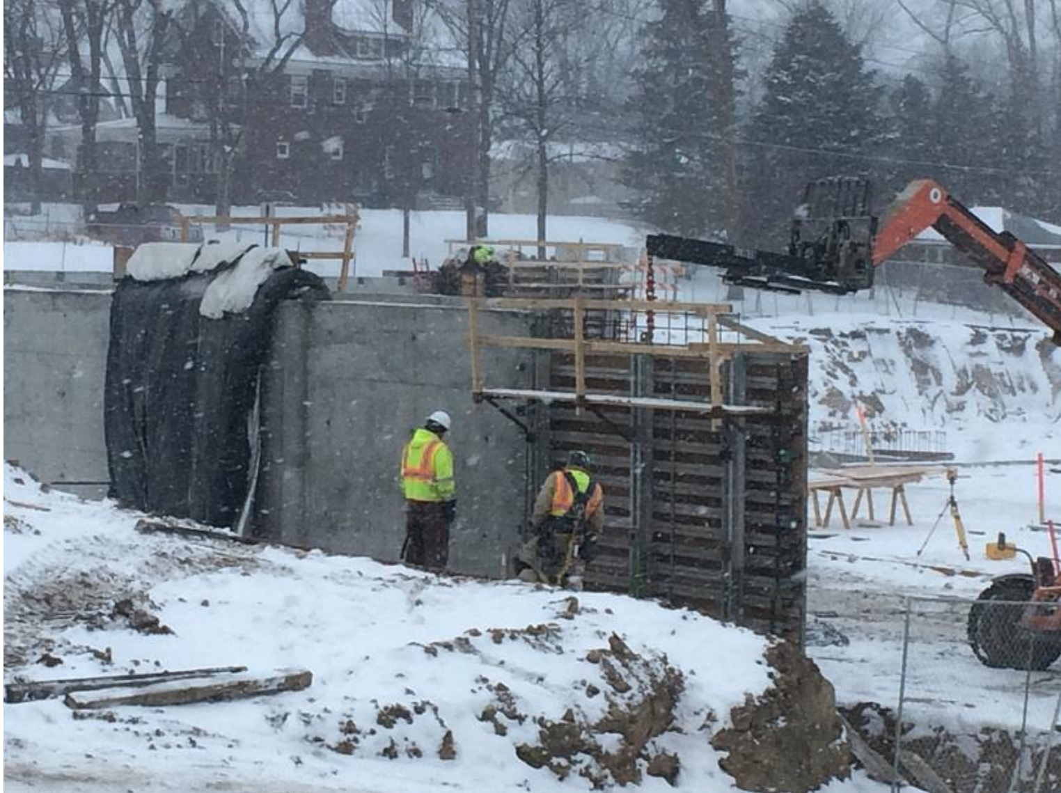
Mcgough setting up for one of the last pours on the tall foundation walls.
